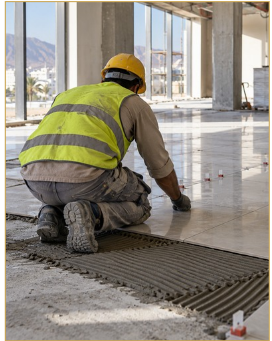
FLOOR TILING INSTALLATION
