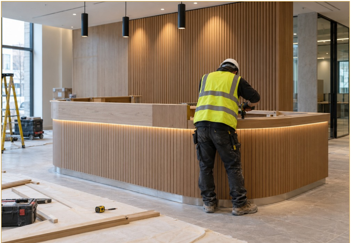
BESPOKE CABINETRY AND TIMBER FEATURES
